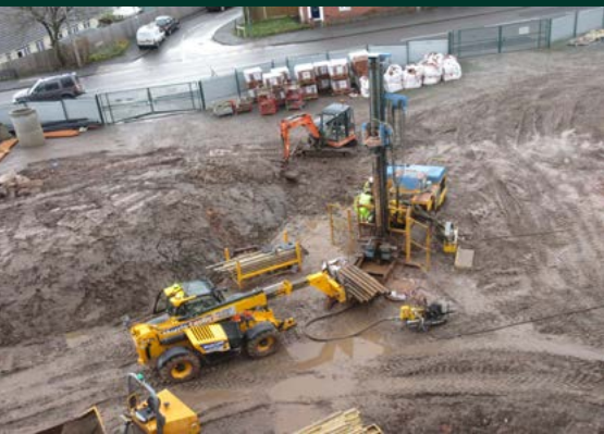
The specialist rig drilling bore holes for the ground-source heat pump. © Historic England
